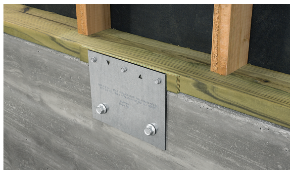
Reinforcement of the connection with the foundation
